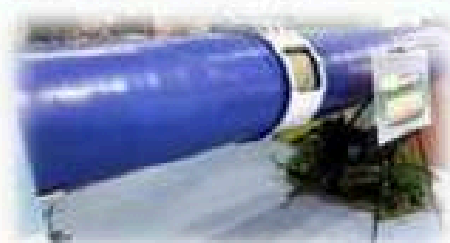
Around the Pipe
